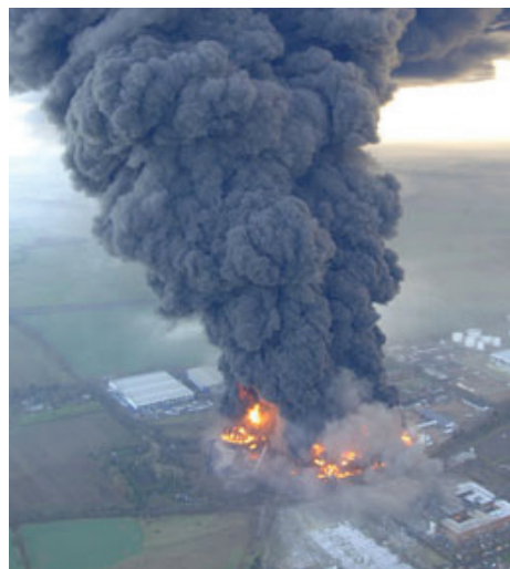
The Buncefield fire (photo: Chiltern Air Support Unit)
