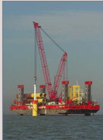
"Jumping Jack" pile driver
