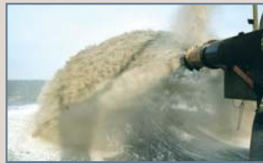
Figure 2. Spreading gravel over the Roughs Tower Spoil Ground
