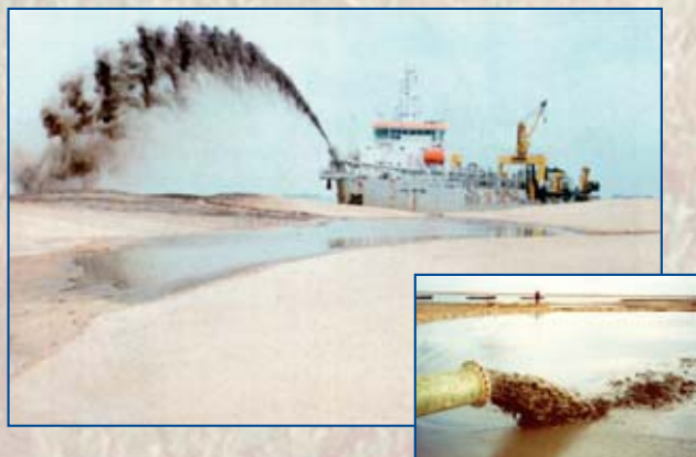
Figure 1: Intertidal recharge of fine-grained dredged material by rainbowing and direct pumping (inset)
