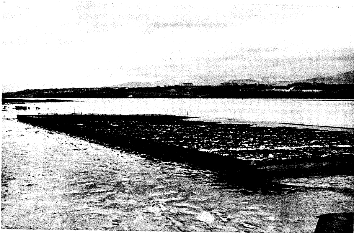
Figure 6(B) The GRP fence enclosing 800 m 2 of mudflat at the Menai Strait: the enclosure contained about 5 tonnes of seed mussels when this photograph was taken in January 1978.
