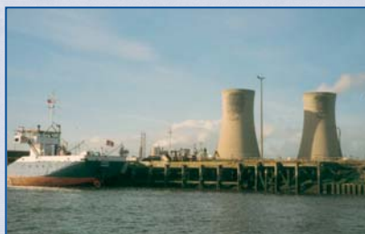
Figure 2 A typical site in an industrialised estuary in the UK.
