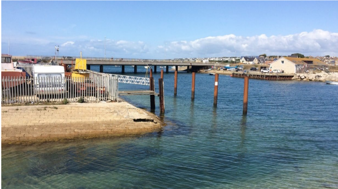
Figure 5. Ferry Bridge with East Fleet lagoon in the background
