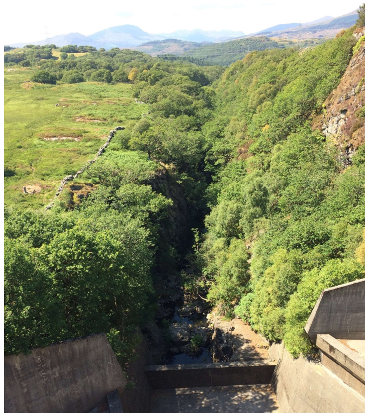
Figure 10. From Maentwrog Dam looking along the River Prysor
