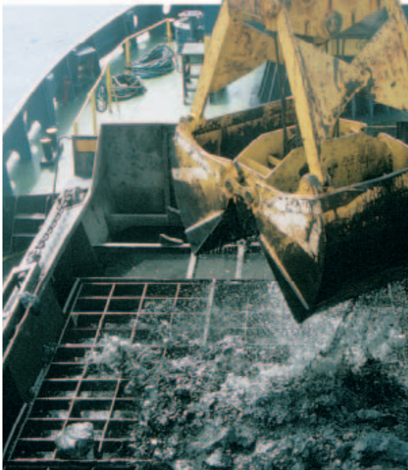
Harbour maintenance dredging
