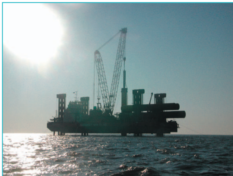
Construction work underway at the Scroby Sands windfarm off Great Yarmouth
