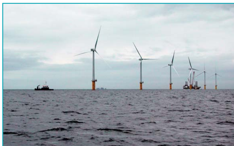
Construction of North Hoyle windfarm, off Rhyl, north Wales
